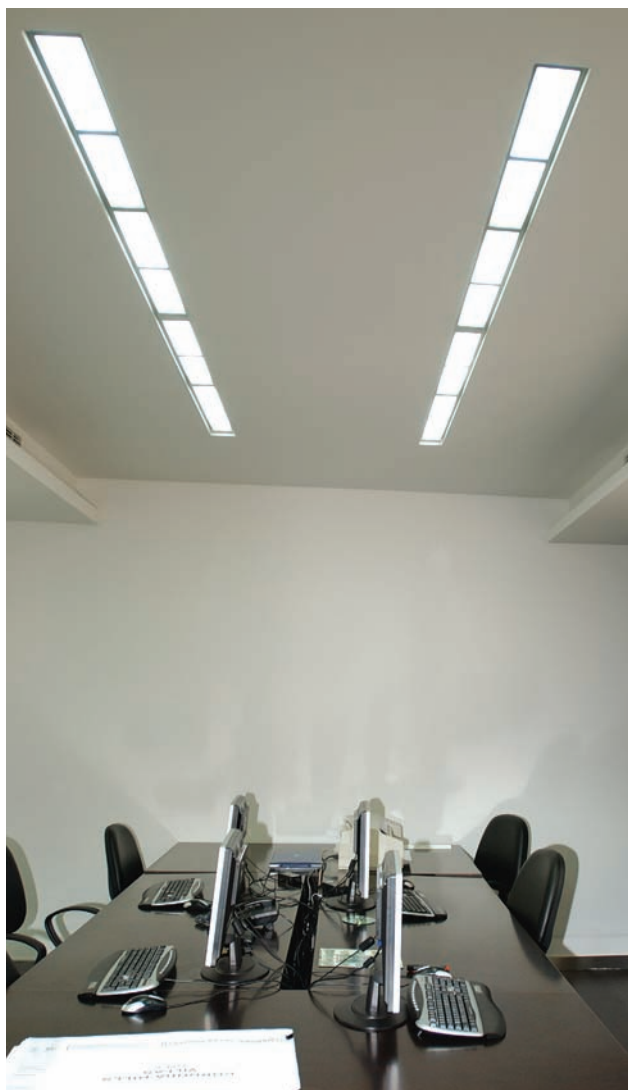
ML 5311-GR Linear luminaire with 2x36W T8 lamps and metallic grill
